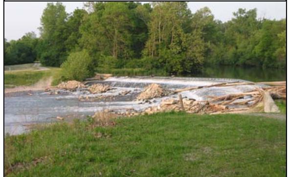
Diversion Dam on the Mad River
