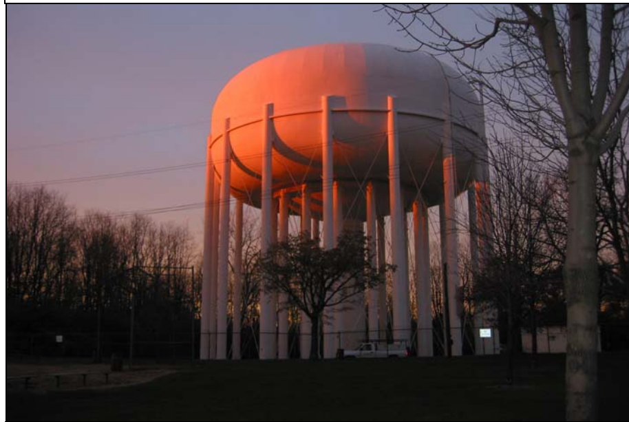
Distribution Storage Tank
